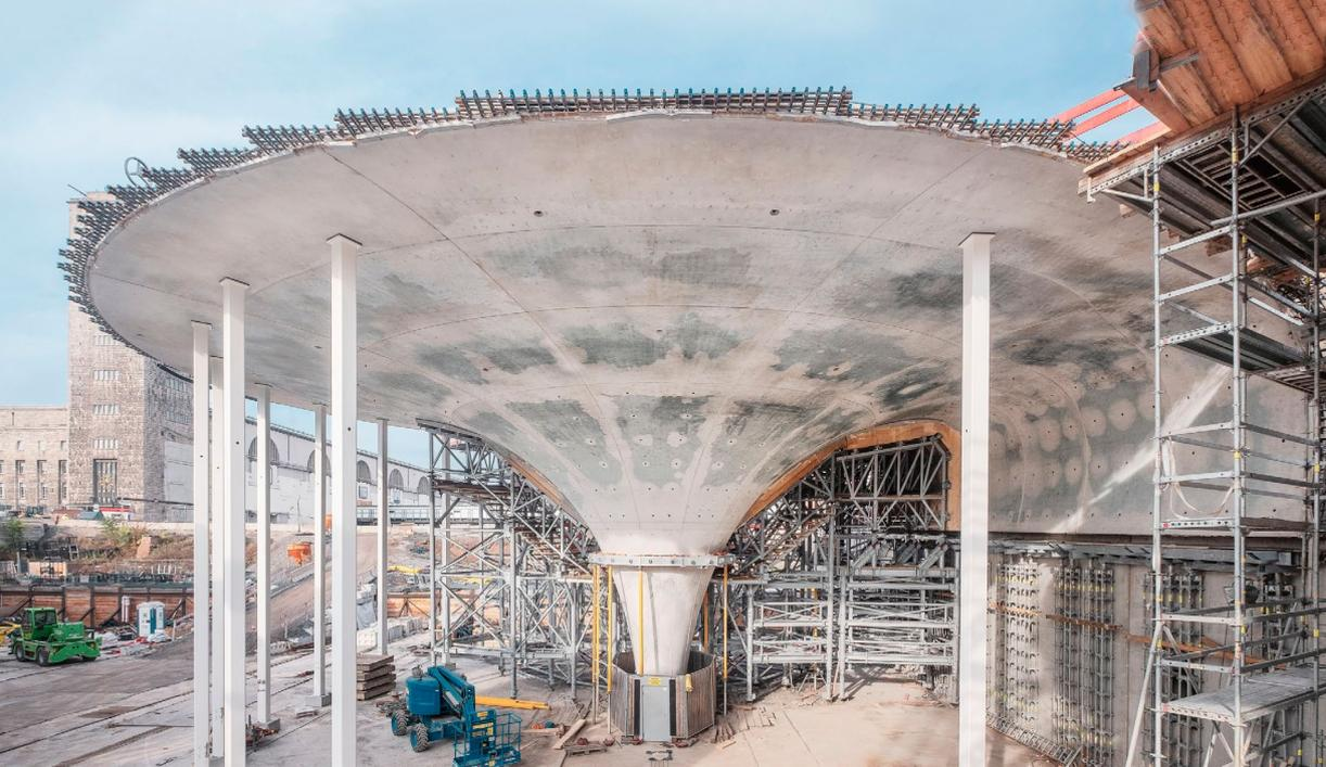
Concreted cup support for the platform hall of the new Stuttgart underground station.
